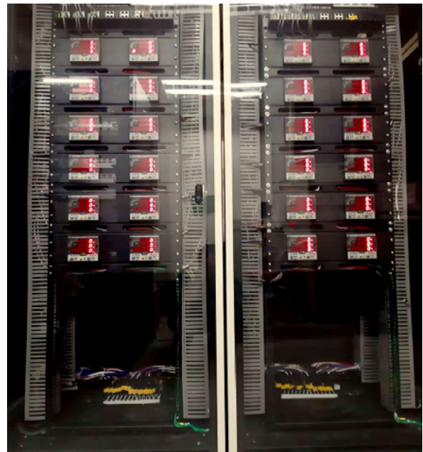
PM175 Substation Installation
